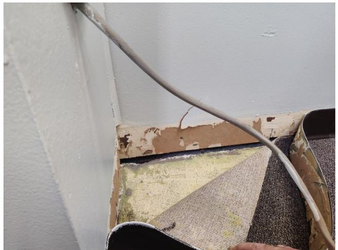
Figure 14: Area where interior wall is separating from floor plate.
