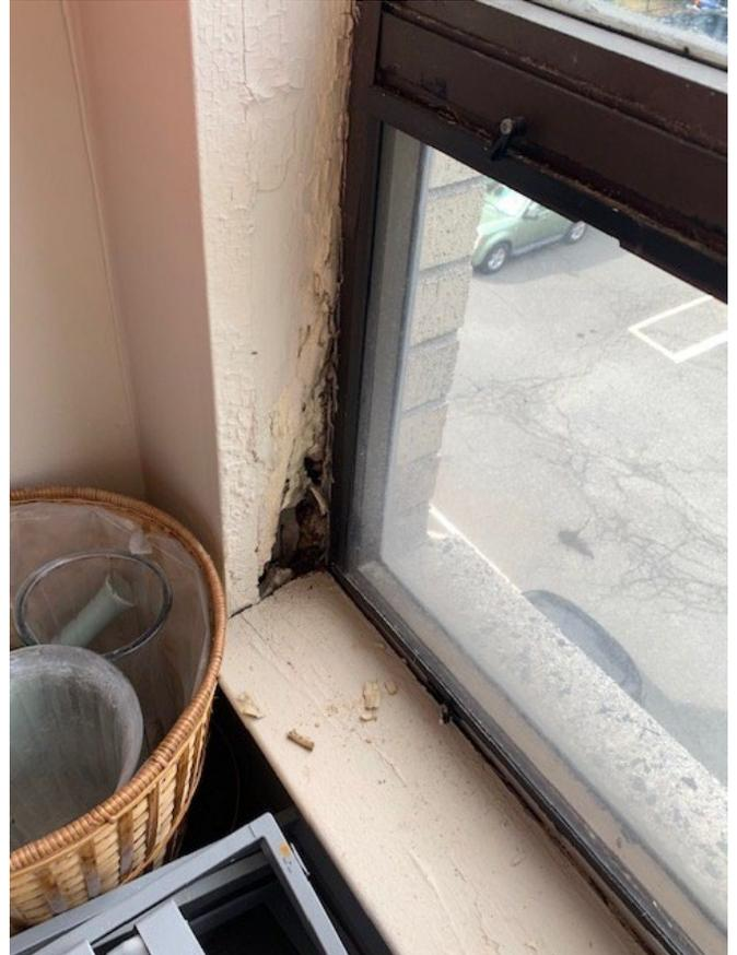
Figures 17a and 17b: Damaged windows.
