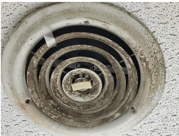
Figure 13: Mold-covered air vents in municipal office.
