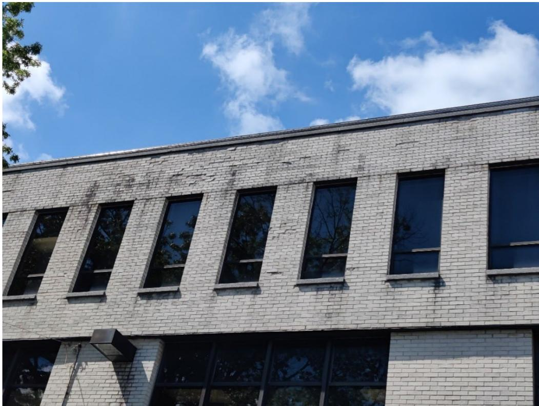
*Figure 19 Area where brick facade is falling off building facade.*
