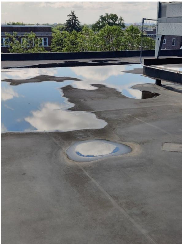
Figure 11: Ponding water on roof.
