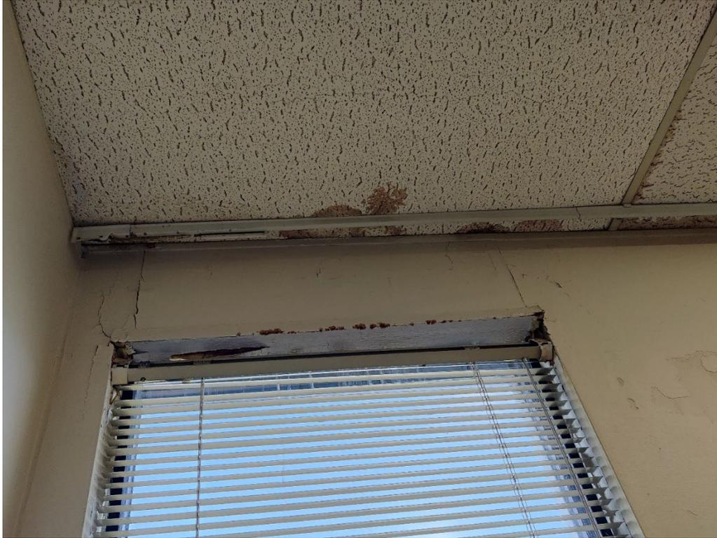
Figure 15: Damaged windows and ceilings in municipal building office.
