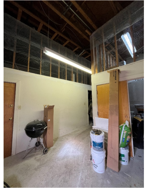
Figure 30: Interior of garage storage areas
