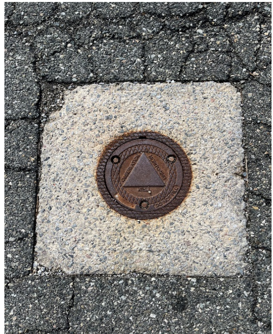
Figure 21: Groundwater contamination observation well
