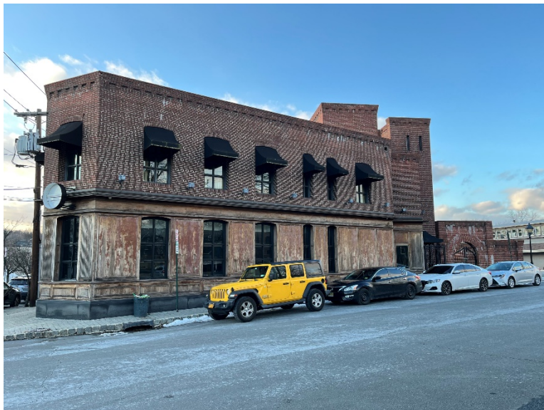
Figure 38: Exterior of 2 Erie, detailing original portion of structure.
