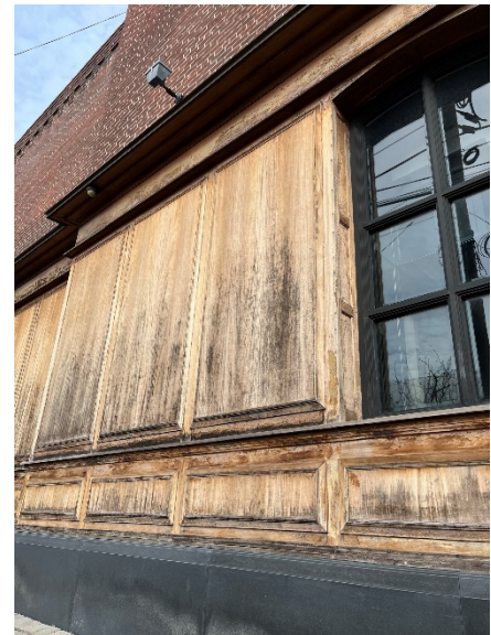
Figure 39: Wood paneling applied to first floor exterior
