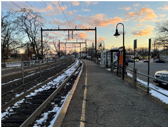
Photo 9: View east up Walnut Street platform
