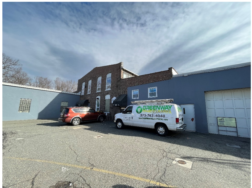
Figure 19: Garage spaces and light manufacturing uses at the pinch point as viewed beside tributary
