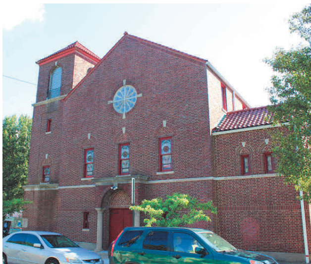
Union Baptist Church (12-14 Midland Avenue, built c. 1930)
