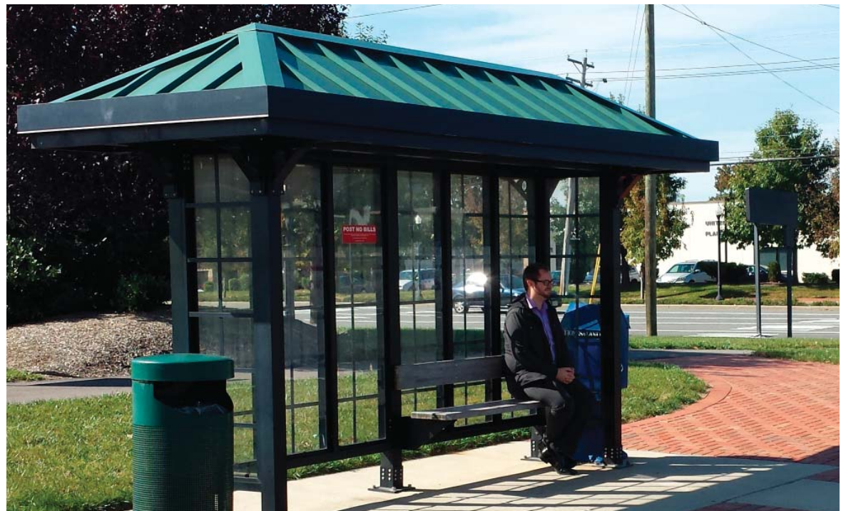
Bus shelter with increased visibility for transit users and bus drivers
