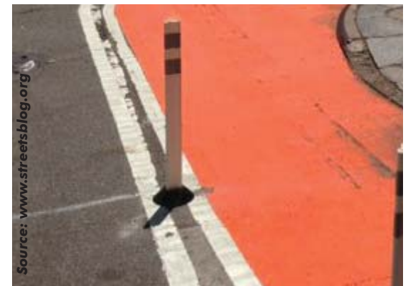
Painted curb extension to assist in guiding drivers with the shift and reduce the perceived road width
