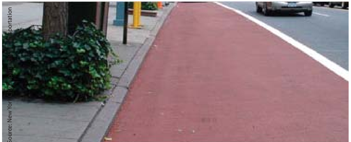
Highlighting bus stop areas with pavement markings will assist with stacking, loading, and help to calm traffic by distinguishing bus pull-offs from parking and travel lanes
