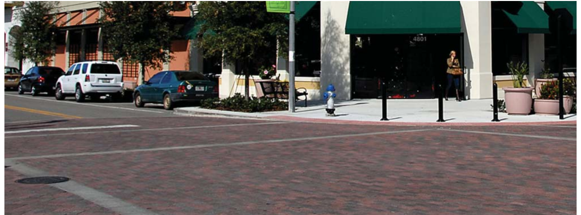
Textured pavement and curb bumpouts
