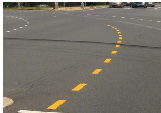
New lane guides to assist in guiding drivers with turning movements
