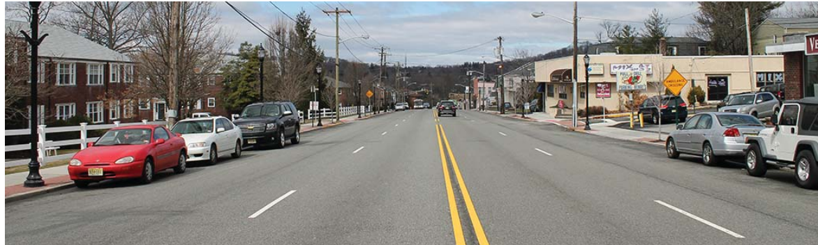
Unmarked parallel parking and four travel lanes on Bloomfield Ave near Church Street in Verona. The perceived road width can encourage higher speeds in some areas in the corridor.
