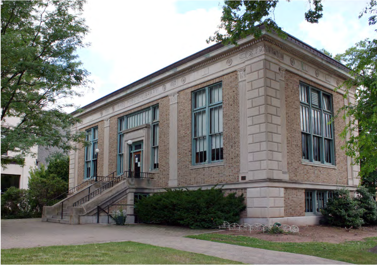
Bellevue Avenue Branch Library (BAB) in 2016, looking NW .
