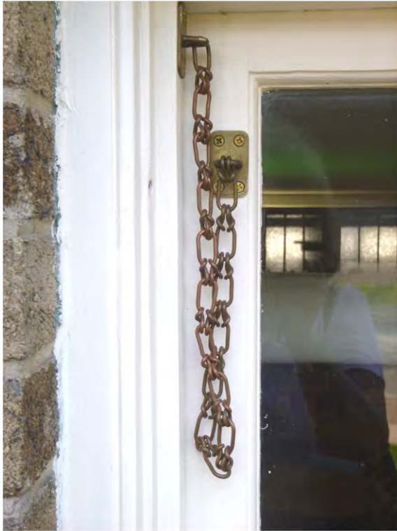
Detail of restored original "weldless" chain on re-installed hopper windows at the lower level children's room, looking W (August 2018).
