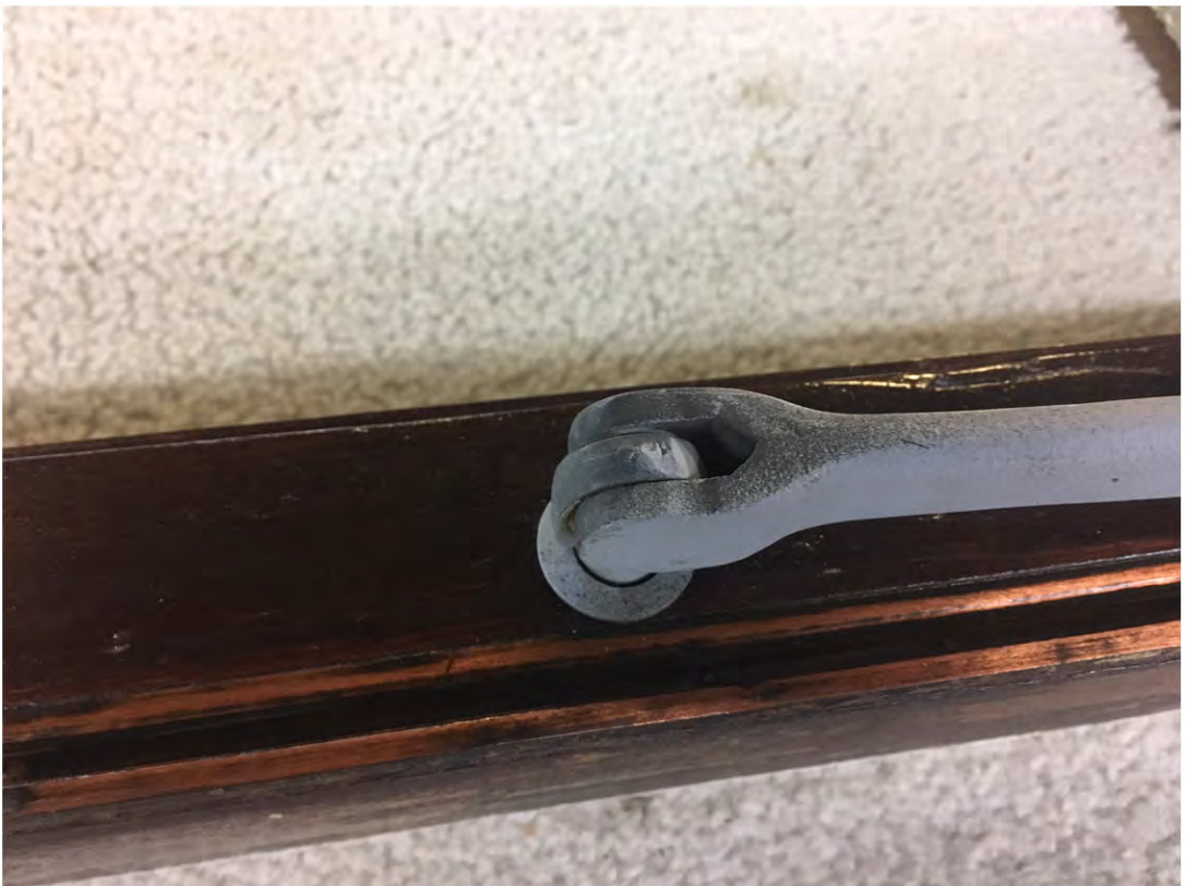
Detail of cleaned and primed lever arm and eye of thru-bolt at Dell-Tech Studio (2018).
