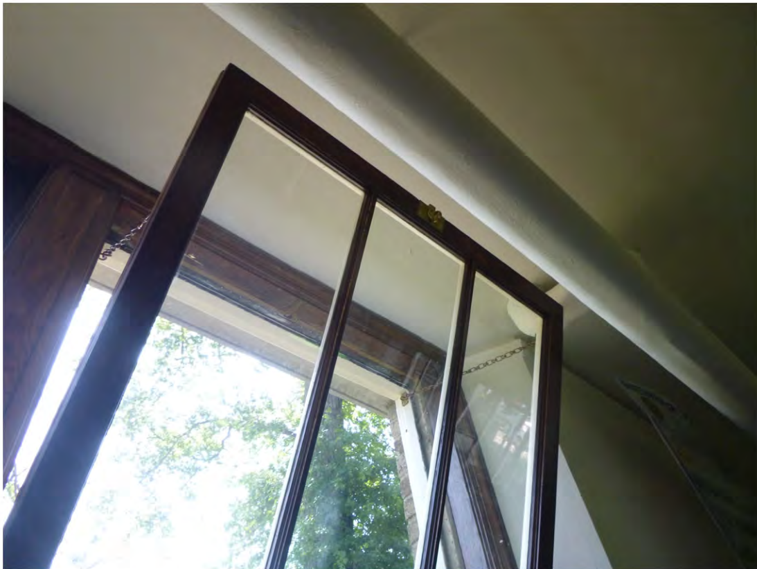
Restored hopper window held in open position by sash chain, east facade (August 2018).
