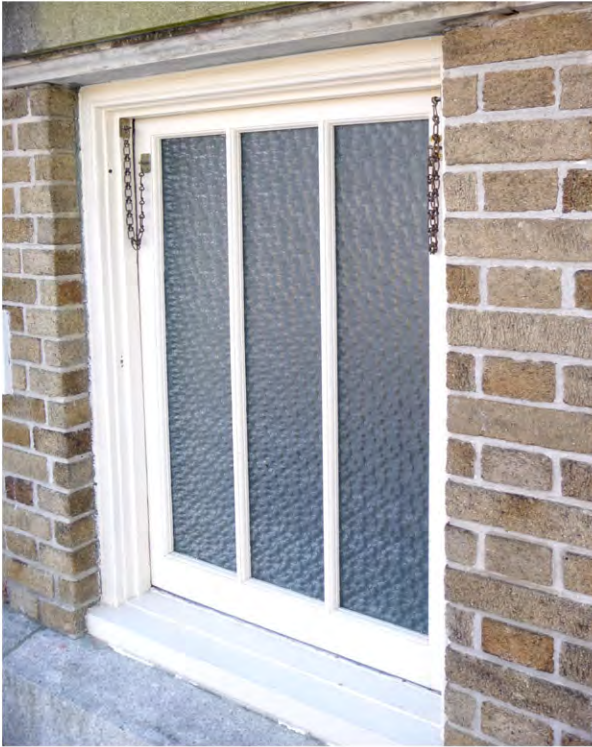
Restored hopper window with replacement obscuring glass, lower level lavatory, looking NE (August 2018).
