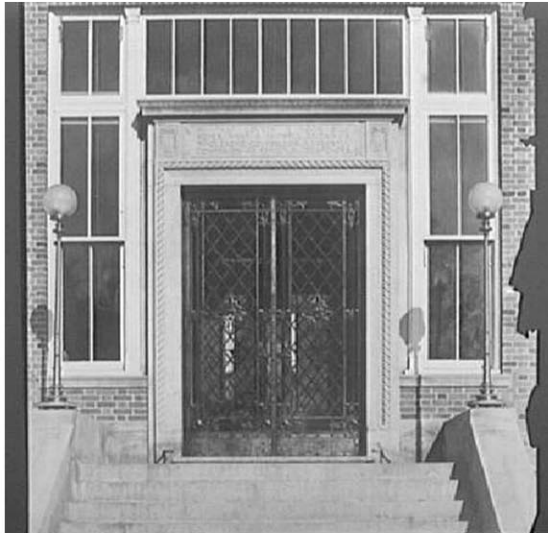
Main entrance on Bellevue Avenue ca. 1915, looking N. The Austral lever arms on lower sash are shown painted to match sash color.
