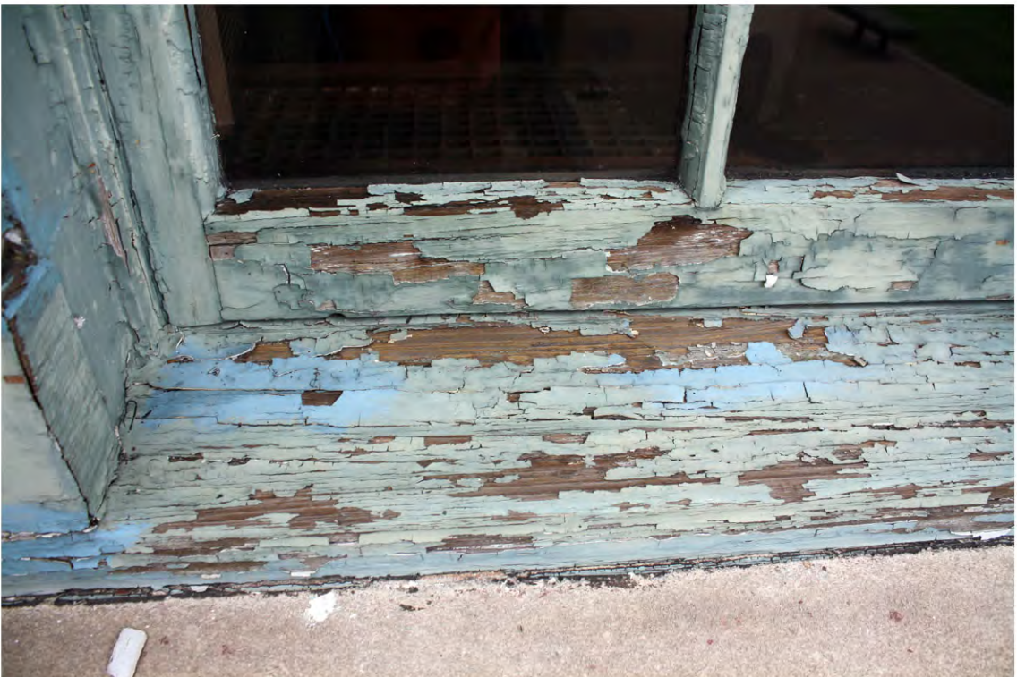
Detail of deterioration on sill at main facade, looking N. .
