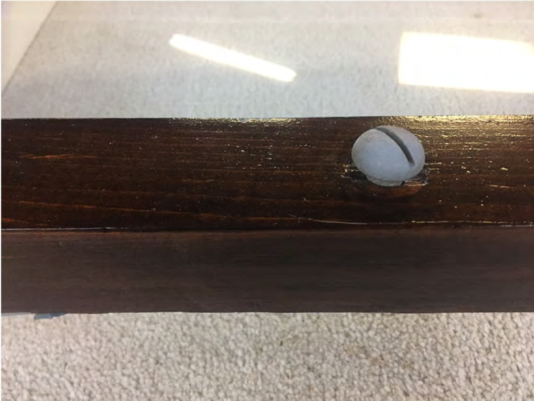
Detail of thru-bolt that holds the lever arms to the sash (at Dell-Tech studio, 2018).
