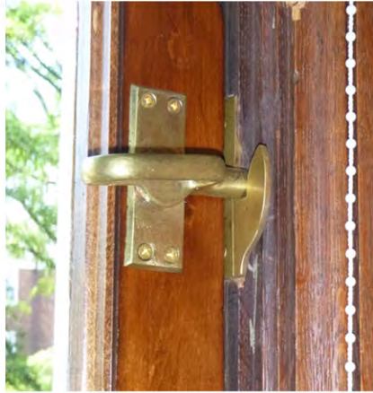
Restored interior sash latch and latch plate (August 2018).
