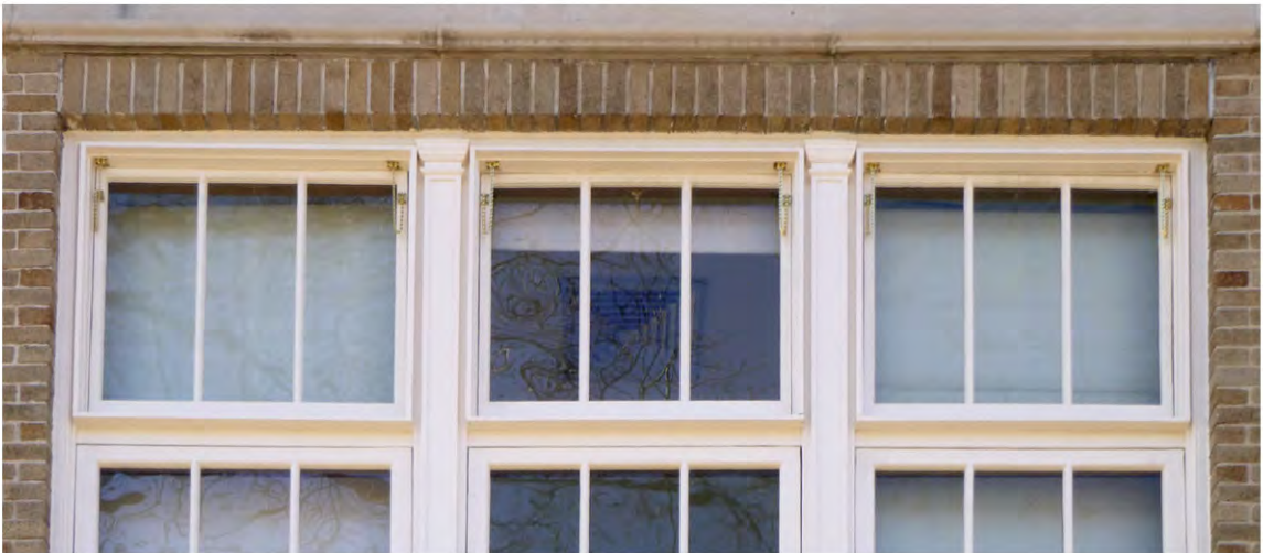
Restored transom windows with replacement chains after installation, east facade (August 2018).
