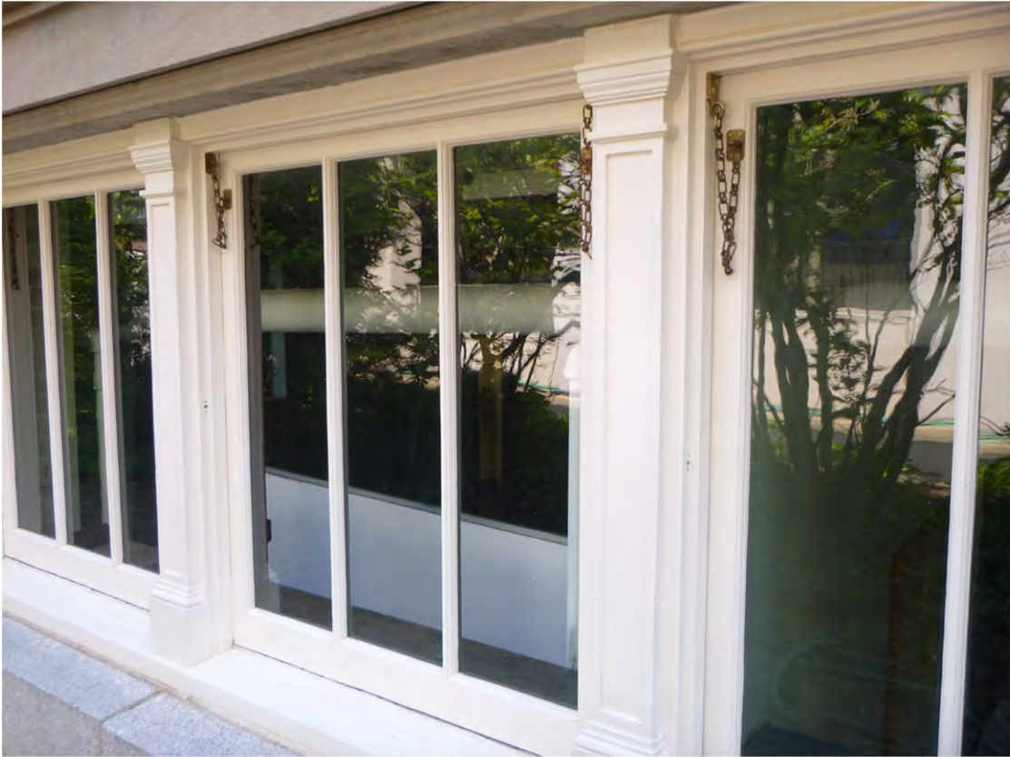
Restored hopper windows with original chains at the lower level children's room, looking SW (August 2018)
