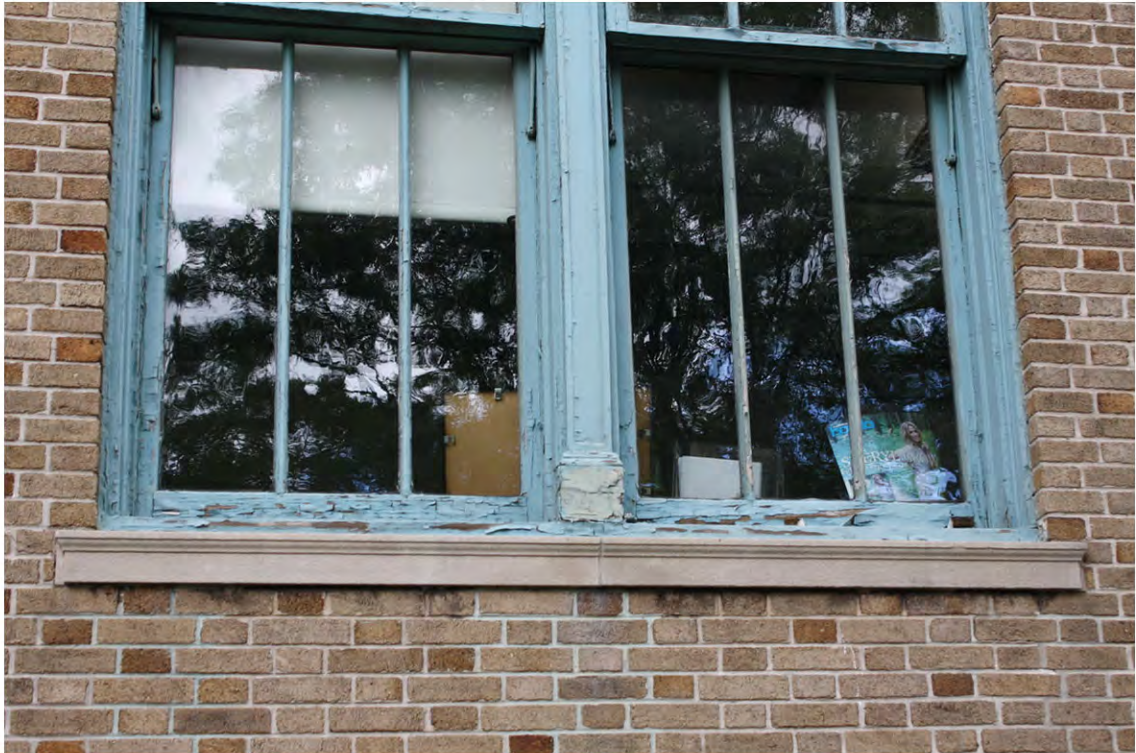
Library windows on south facade in 2016, looking N, showing level of deterioration.
