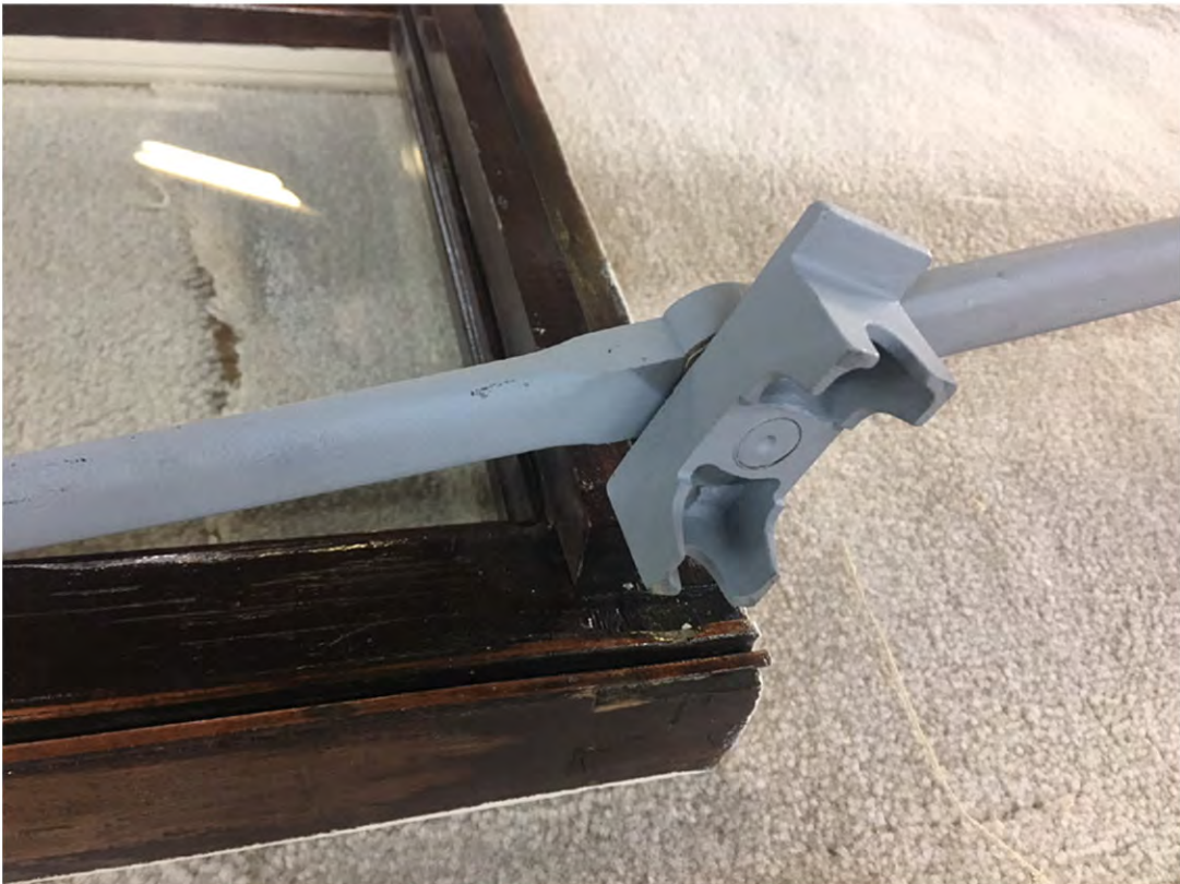
Detail of cleaned and primed bracket on lever arm for mounting onto jamb (at Dell-Tech Studio, 2018).
