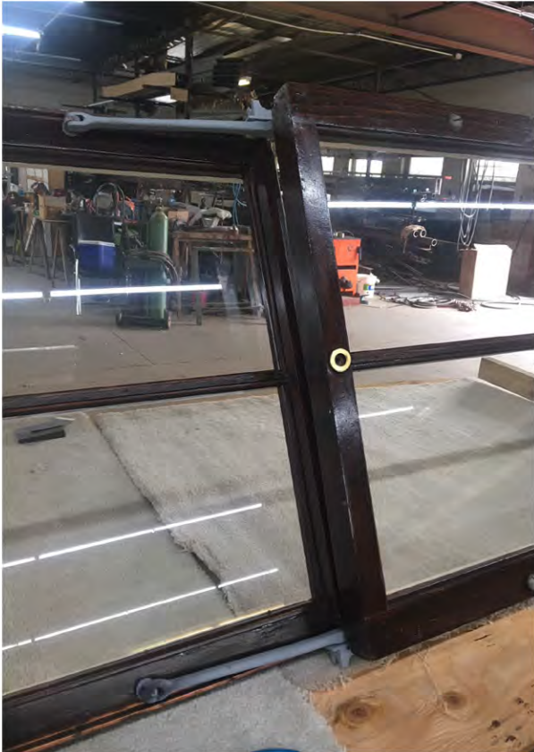
Detail of interior of Austral window assembly, with upper sash at left, lower sash at right, with restored brass grommet around hole for the hook that operates window movement (at Dell-Tech studio, 2018).
