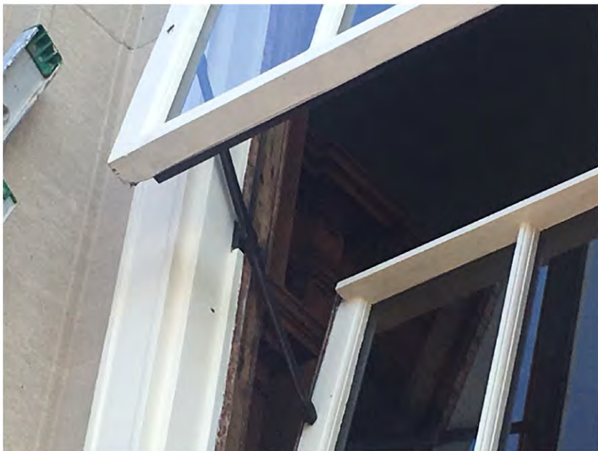
Test operation of Austral windows (May 2018).
