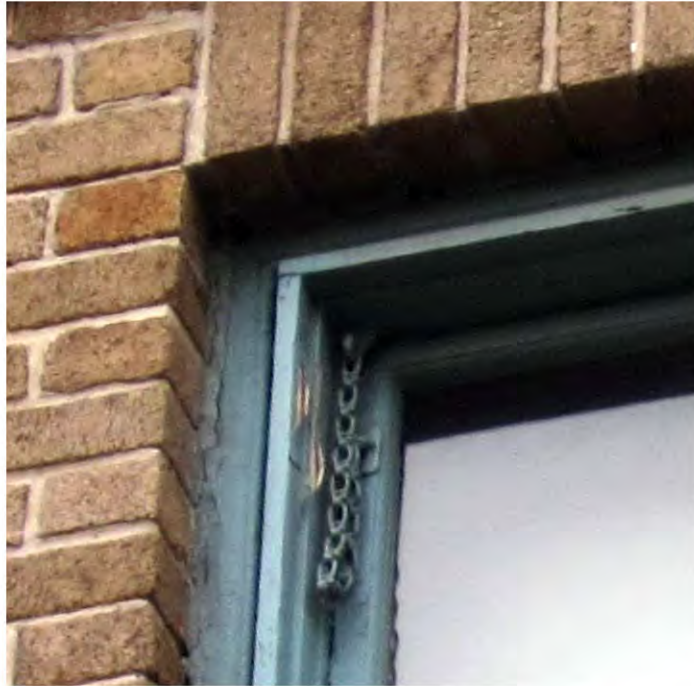
Typical condition of painted sash chains in 2016.
