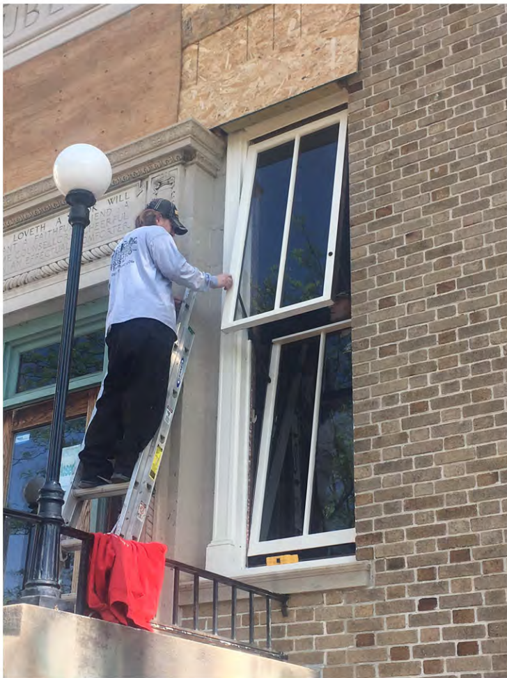
Test installation of rehabilitated Austral window on main facade (May 2018).
