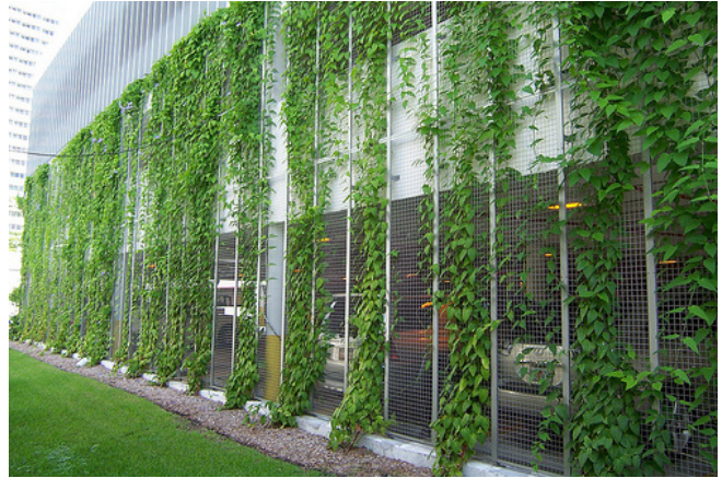
B.8-07: A planted green screen applied to a parking structure shades the interior, screens the deck structure, and visually softens the spaces around the deck.
