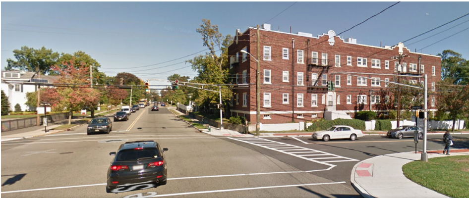
B.6-07: The intersection of Grove Street and Glenridge Avenue, looking north. A 3-1/2 story apartment building at the northeast corner of the intersection provides a fine example of Midrise design, using contrasting masonry to define the building base and enliven the roof line.
