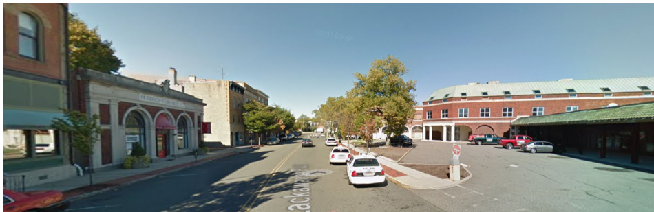
B.6-05: Next to the former Train Station Waiting Room, looking north along Lackawanna Plaza, also known as Israel Crane Way. The Terminal Shed, with non-original enclosures beneath, is seen on the right, terminating in a 2-1/2 story brick office building built in the 1980's. The west side of Lackawanna Plaza features a variety of building styles and uses. The overall vista culminates in Israel Crane Park.
