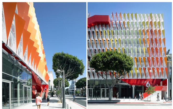
B.8-09: A repetitive system of three-dimensional elements is a powerful way to screen a parking deck. Depending upon the viewing angle and the use of color and form, the screen will change appearance from different vantage points.
