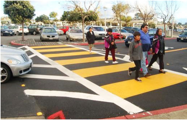
C.13-03: This wide speed bump doubles as a pedestrian path cutting through a parking area. Shallow asphalt ramps, diagonal striping and broad colorful bands highlight the walking zone, ensuring that drivers are both physically and visually aware of the path.
