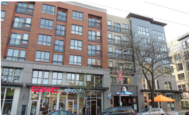
A.3-02: Discouraged: The base-middle-top facade strategy is rooted in traditional design, as are varied setbacks and cornices. When the materials and details of local design examples are ignored, however, new buildings can appear generic and cookie-cutter.
