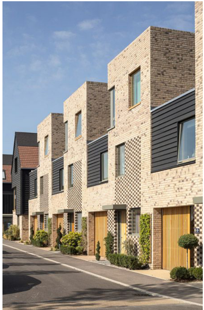
C.4-09: In lowrise construction, often used to transition from midrise masses to the scale of adjacent single family residences, smaller repeated masses are effective when articulated with materials and textures that echo traditional design.
