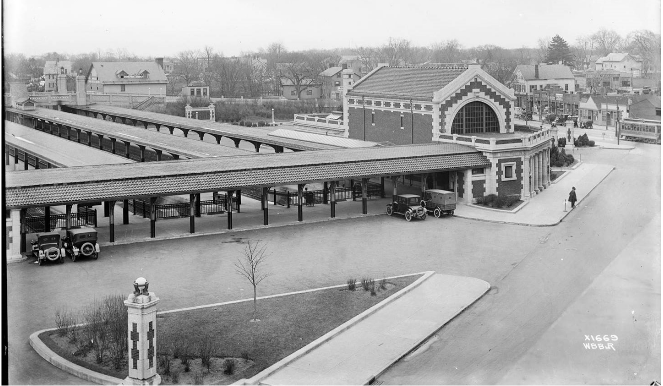
B.3-04: The Lackawanna Train Station, as seen c. 1915, soon after its completion. The Station has been altered over time, but this overview makes it possible to imagine how it functioned originally. In the foreground is the open-air Terminal Shed, the covered area where the train tracks and waiting platforms ended. Beyond the Terminal Shed are the long open-air Platform Canopies (integrated into the existing Lackawanna Plaza structure in the 1980's). The Platform Canopies consist of steel columns with flared steel beams supporting cantilevered concrete roofs. At center right is the Waiting Room structure, where passengers could buy tickets and walk directly outside, under cover of the Terminal Shed and the several Platform Canopies, to the appropriate train platform. The brick Horse Watering Trough is partly visible, center left.
