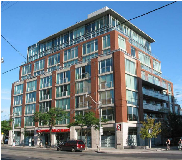
A.5-06: Discouraged: Uniform setbacks on all sides of a building threaten to create a pyramid effect, highlighting overall mass rather than minimizing it. Where upper stories of a new midrise building will be visible from several directions, this must be avoided.
