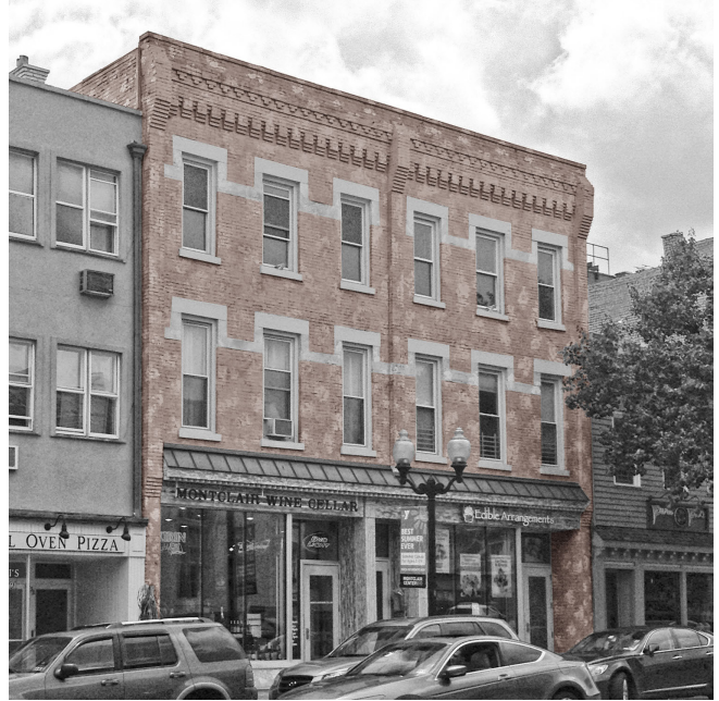
B.4-05: Buildings do not require expensive carved stone or molded masonry to create a contextual facade. Brick pilasters, draped lintels and a corbeled brick cornice at 440-444 Bloomfield Avenue
