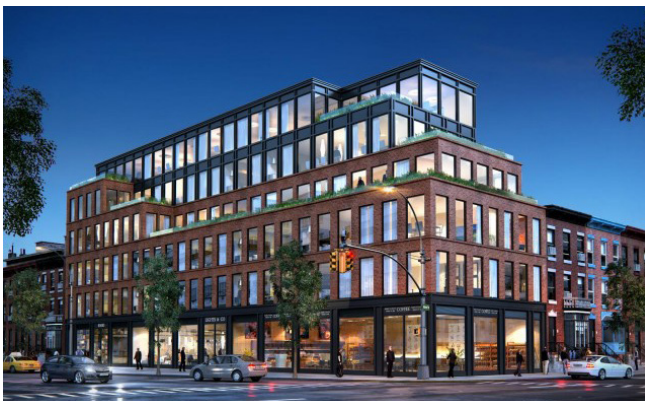
A.5-02: Encouraged: Multiple stepbacks allow a six-story building to continue a three-story streetwall established by its older neighbors, with its upper three stories progressively reduced in visibility.
