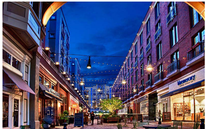
A.2-02: Encouraged: Shoulder-to-shoulder buildings facing one another across a street or public plaza create a sense of enclosure and safety, and transform public spaces into comfortable "outdoor rooms" that invite lingering by residents and visitors.
