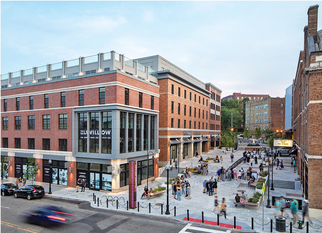
B.5-05: In mixed-use design, the requirements for different kinds of programming - ground-floor retail, upper-story residential, screened parking structures - lend themselves to form-making that breaks down larger masses. Above left, at the Seymour Street redevelopment project in Montclair's town center, transparent bases, uniform middle stories, distinct cornices, and top-story stepbacks reduce the apparent scale of a trio of new 5 story buildings. A canted metal screen on the new parking garage, middle right, provides an effective modern foil for the buildings and plaza.
