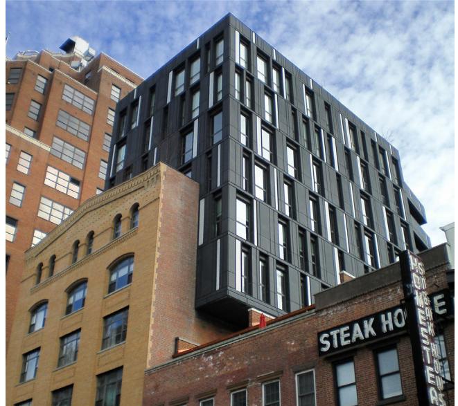
C.4-13: Inspired by its blocky neighbors with their punched openings, this addition steps back from the street, projects to the side, and uses metal as a contrasting material. It preserves its historic base while asserting its role in redefining the site's use from commercial to multi-family.
