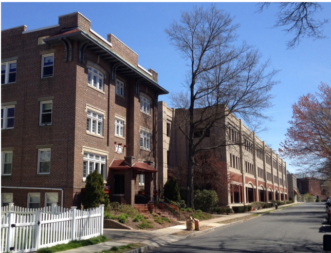
B.8-06: Extra care is taken to ensure that the Crescent Deck is respectful to the immediate multi-family housing building. The buildings share a very similar scale, and precast window details are employed by both structures.
