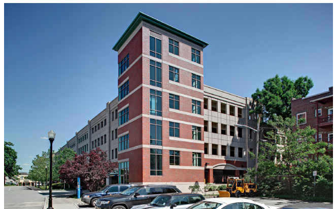
B.8-04: The Crescent Deck picks up on architectural cues - massing, detailing, material use - from neighboring traditional multi-family housing. The deck’s location provides car queuing and some relief from adjacent heavily used thoroughfares.
