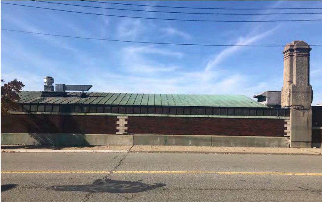
Grove Street stair and North Pylon
