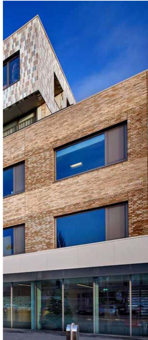
C.9-01: The base-middle-top composition of traditional “Main Street” facade design can be creatively interpreted in order to produce an effective midrise design.
