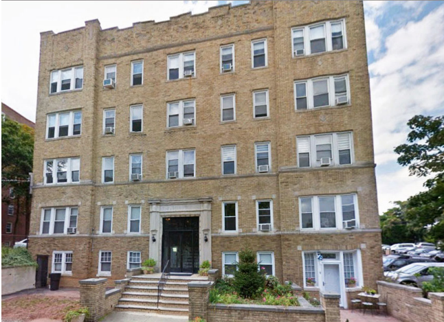
B.5-04: Multi-family apartment buildings along the edges of Montclair's Town Center display what a base-middle-top strategy can look like when not employed by a mixed use building, as typically seen along Bloomfield Avenue. Shallow massing projections divide the building into vertical bays, breaking down the scale of the four-story structure. Stone framing the central entrance matches a stringcourse and the window sills, unifying the composition.
