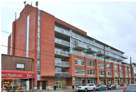
C.4-17: A three-story brick and storefront base (right) ties into the existing, lower context while a vertical brick mass (left) announces the transition to a taller re-zoned area. Stepbacks from right to left and glass “infill” zones mitigate overall mass.
