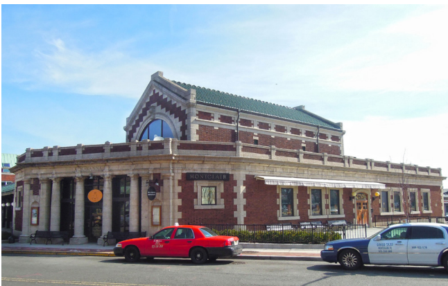
B.2-04: Although no longer serving its original function, the 1913 Beaux-Arts Lackawanna Train Waiting Room's entry collonade, distinctive window surrounds and matching quoining, bold parapets, and arched thermal windows create a grand impression.
