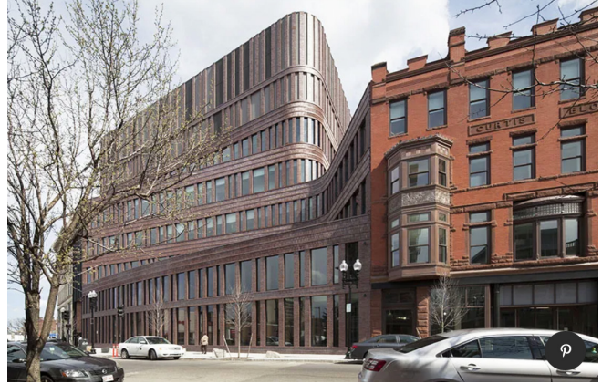
A.5-03: Encouraged: Stepbacks must be combined with clear form and detail to work effectively. To ally itself with an older building (at right), the above building starts with a tall glazed base, steps back with a middle facade parallel to the older structure, and adheres to a reductive, historically-compatible palette of glass and metal.
