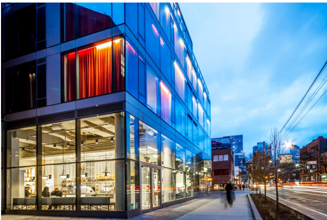
C.4-11: Reductive Modern design, if respectful of the storefront culture that fuels the walkable "Main Street", is no less effective than historic design. Thin floor plates and finely detailed glazing on upper floors produce a delicate lowrise design.
