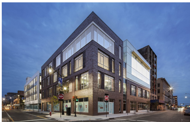
C.4-07 Historical material and style, such as brick and industrial openings, can be combined with new materials and expanded glazing to create a building suited for modern functions without seeming out of place in a walkable town center.
