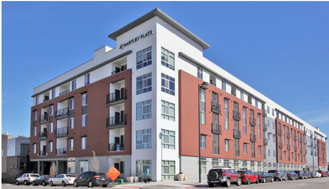
A.3-01: Discouraged: Brick is often employed across the country to imitate existing traditional architecture. When applied like wallpaper to a bare box, however, brick loses the depth and character associated with its historic precedents.
