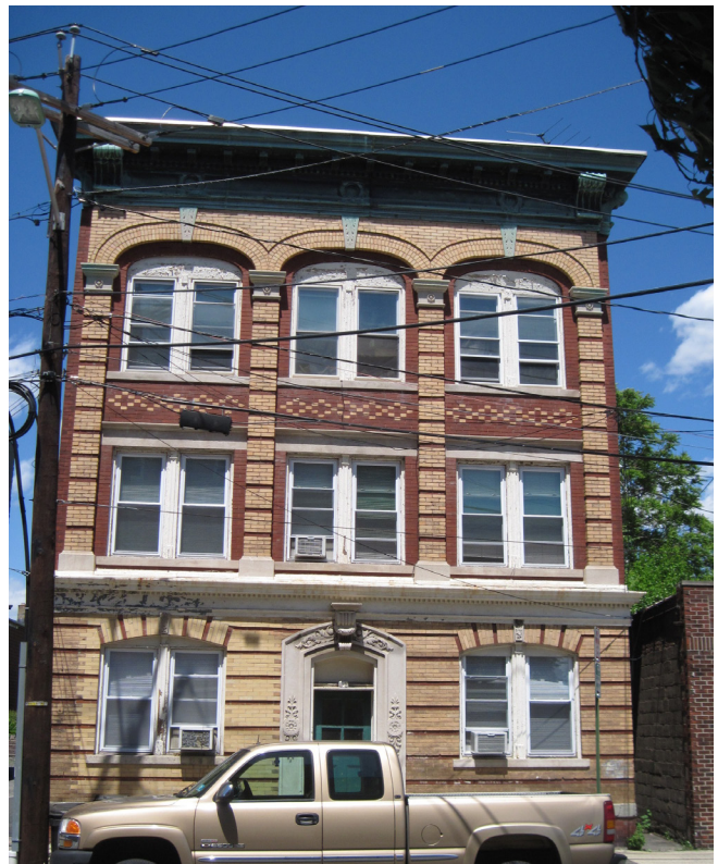
B.4-02 (above): While lowrise, these 3-story apartment buildings on Glenridge Avenue, near the redevelopment area, demonstrate different strategies for bringing visual interest and variety to a familiar building type. It is not hard to imagine modestly “growing” these structures by adding a fourth floor in contrasting form or material, or by stepping back the additional floor.
