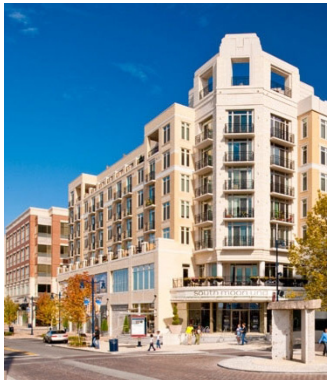
A.5-04: Encouraged: A prominent corner transition employs a deep entrance canopy and third-story stepbacks on the side to create a welcoming streetscape and an architectural rhythm easily legible to pedestrians.
