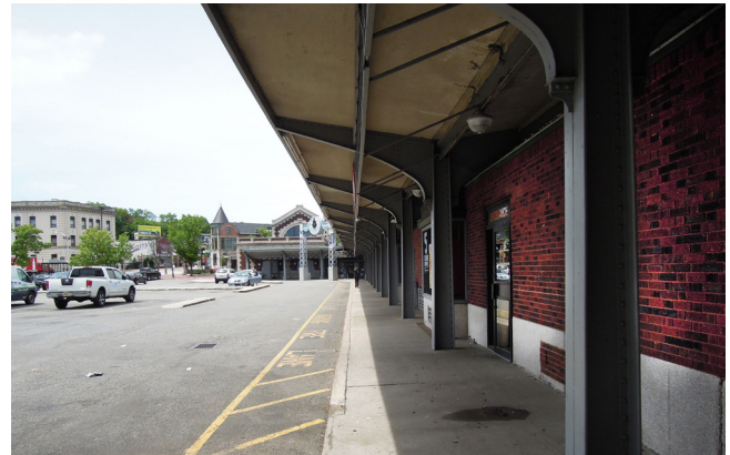
B.3-03: This recent view, comparable to the view above, shows how the 1980's brick wall interrupts the first Platform Canopy, impairing its historic integrity as a free-standing structure.
