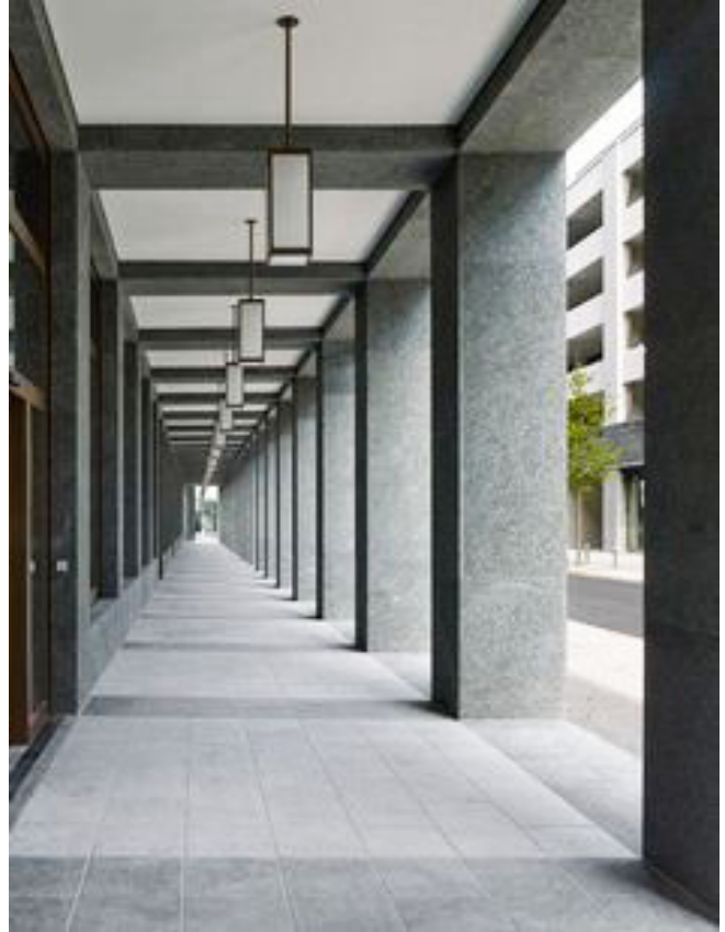
C.13-06: With a simple rhythm of piers on both sides, this long loggia offers the same advantages as a classic arcade. Shallow recesses on one side can serve as art alcoves, promotional display, storefronts, or building entrances.
