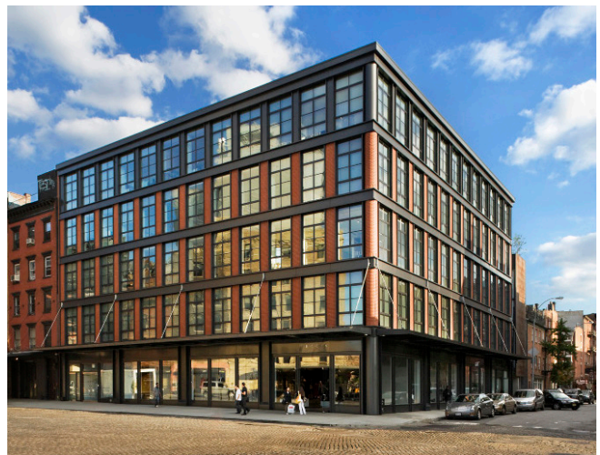
C.4-04: Holding the corner of a block in Tribeca, this transitional design borrows the proportions and materials of nearby historic cast iron loft buildings. In the middle floors, brick piers substitute for cast iron, a nod to adjacent masonry buildings.
