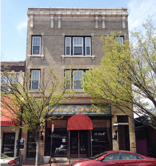
B.4-03: The Louis Harris Building on Park Street is organized into a bold base-middle-top composition using a tall storefront, decorative bands, and individual ornaments. Windows are grouped and spaced to emphasize verticality.
