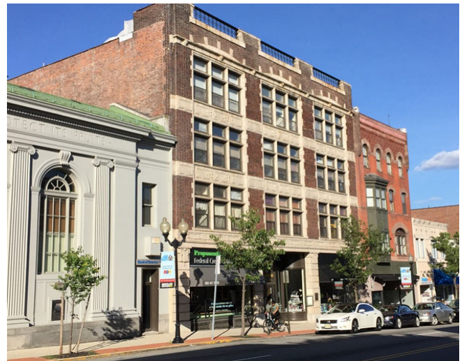
B.5-03: The Madison Building uses grids of varying scales and rhythms in order to reduce its perceived scale. Differences in height and width between it and its neighbors are visible in this photograph, but hardly apparent at the pedestrian level.
