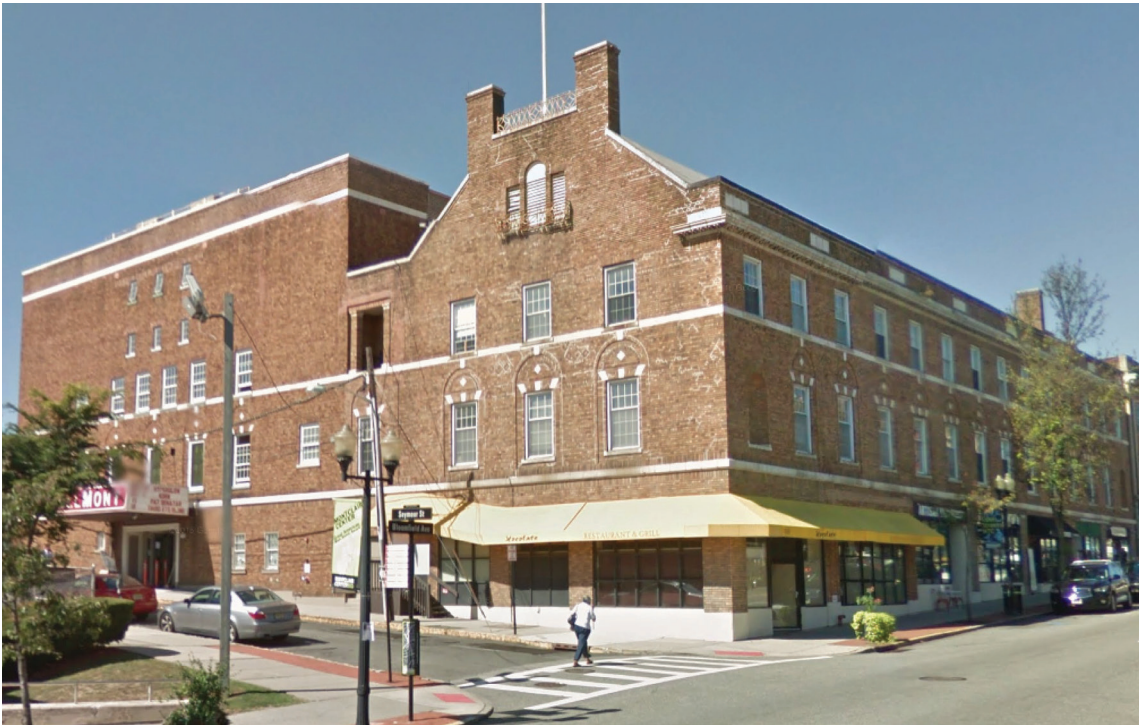
B.4-04: Constructed together, the Wellmont Theater and Kahn buildings share an architectural language but are massed to differentiate themselves and present very different faces along Bloomfield Avenue and Seymour Street.
