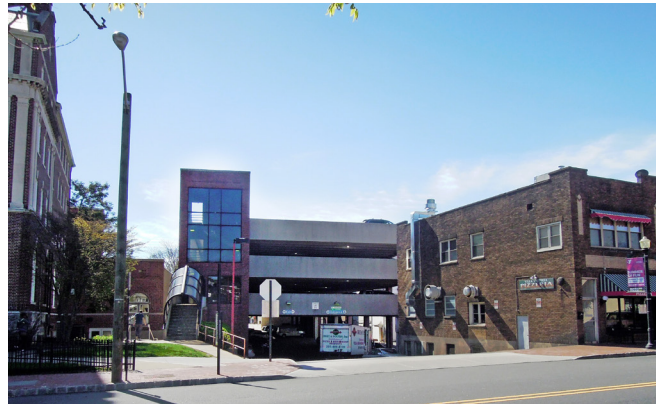
B.8-02: The North Fullerton Deck’s deep setback leaves it hard to find and foreboding. The Deck’s western entry is below grade, making it hard to find. Its eastern entry is close to Bloomfield Avenue, resulting in a cramped approach and increased congestion.
