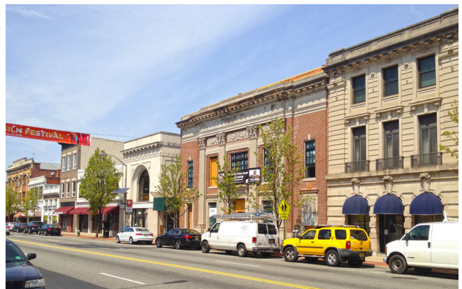
B.2-07: Montclair's Town Center provides numerous instances of well-designed structures of varying architectural style collected in close proximity. This combination of quality and variety is pivotal to the Town Center's built character.
