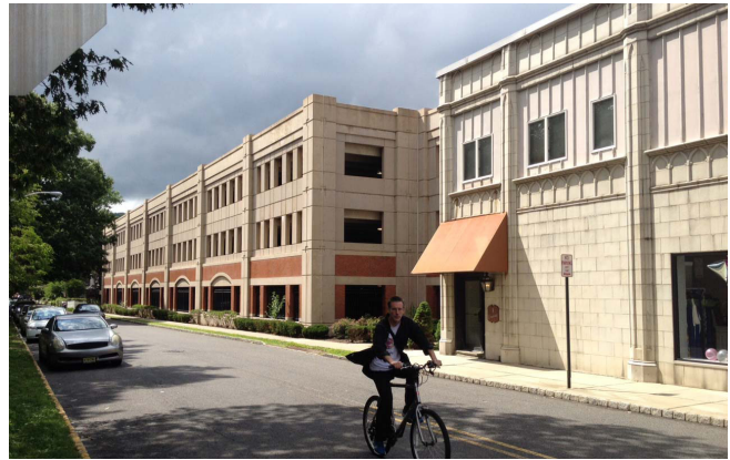
C.13-01: As a visible, free-standing structure, the Crescent Deck is widely appreciated in Montclair for its appearance and generous interior. It blends into its context by picking up on architectural cues from commercial and residential neighbors.
