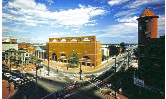
A.3-03: Encouraged: Town Centers need not be frozen in time. Imitating surrounding structures is not required to create buildings that reflect the character of their context. The design of buildings can respond to surrounding architecture through the interpretation and modernization of details. This Portland, ME museum takes cues in form and material from local landmarks.
