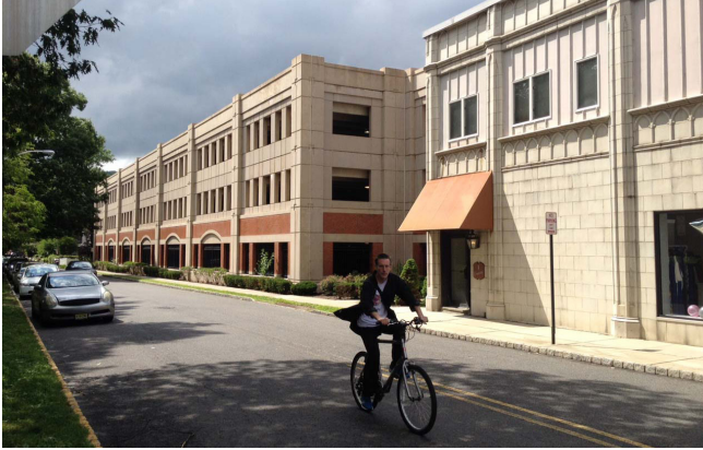
B.8-05: Along The Crescent, the Crescent Deck utilizes the architectural lessons from its commercial neighbors, extending the streetwall and emulating older architecture through modern precast concrete detailing.
