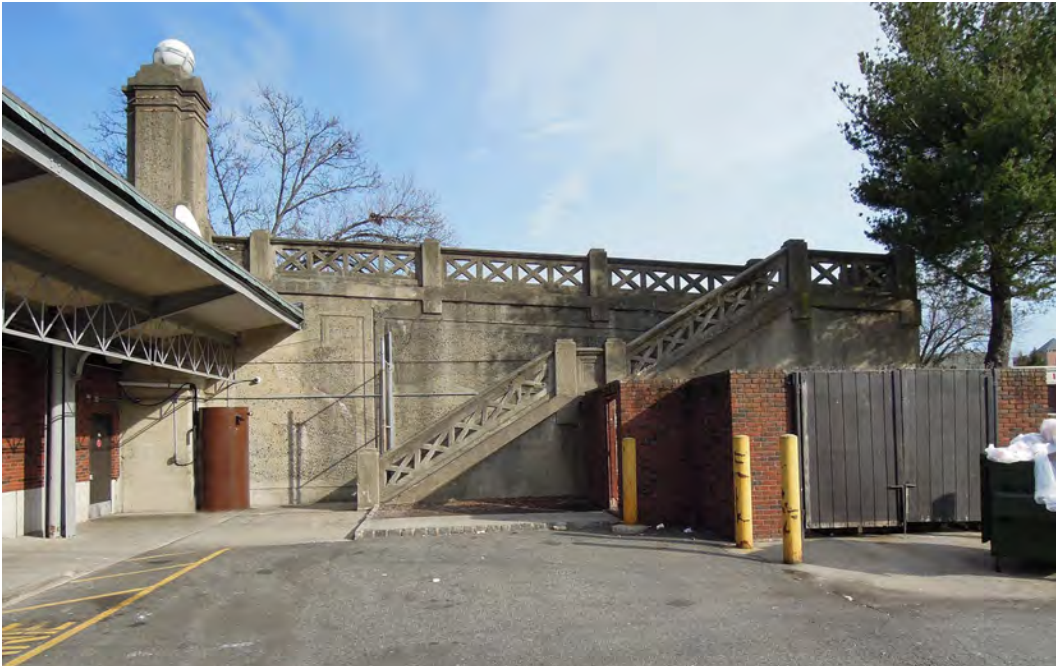
Grove Street stair and South Pylon
