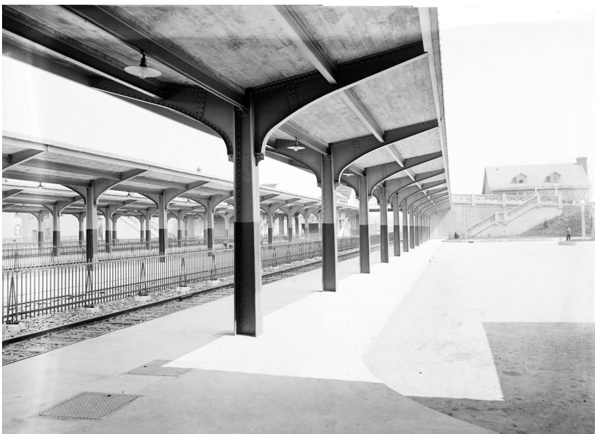
B.3-05: Looking east from the Waiting Room, c. 1915, the Platform Canopy closest to Bloomfield Avenue leads to a concrete stair (partly extant) that brought pedestrians up to the decorative concrete Grove Street bridge. The present-day brick wall facing Bloomfield Avenue (enclosing miscellaneous businesses, including Popeye's), was erected in the 1980's, immediately adjacent to the steel columns of this Canopy. The full concrete canopy remains intact and is visible inside, on the other side of the present-day brick wall.
