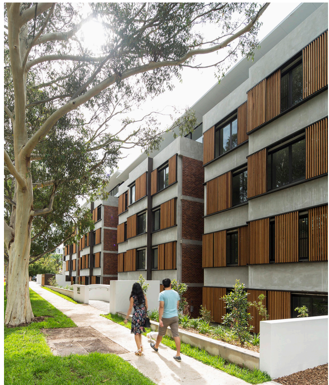
C.4-16: Background fabric doesn’t mean dull. With wood, brick and stucco, these three-story masses, set against a four-story mass, provide an effective, Interpretive Modern transition from a commercial to single-family residential area.
