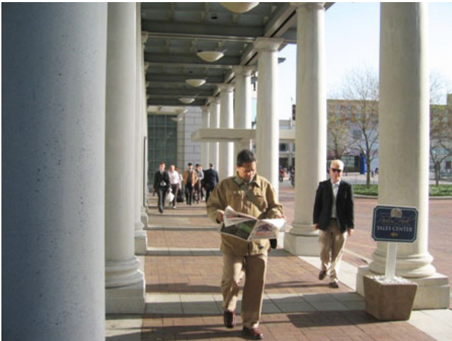
C.13-05: A classic arcade offers a handsome example of an effective, protected passageway. Repetitive columns echoed by simple paving and lighting provide a rhythm that adds interest and human scale to an otherwise lengthy passage.
