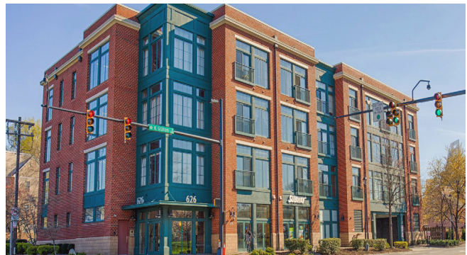
C.7-01: A recessed vertical bay element, similar in width to the building's standard bay, unobtrusively highlights the corner.
