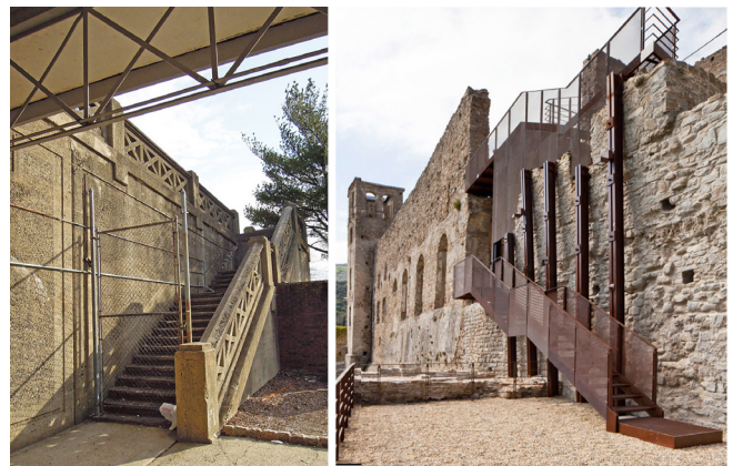
C.12-06: Existing but compromised historic elements, like the remaining Grove Street stair (above left), are excellent candidates for modern interventions that both restore function and dramatize old and new elements, as seen in a new steel stair providing access to a breach in the masonry of an ancient French fortification (above right).
