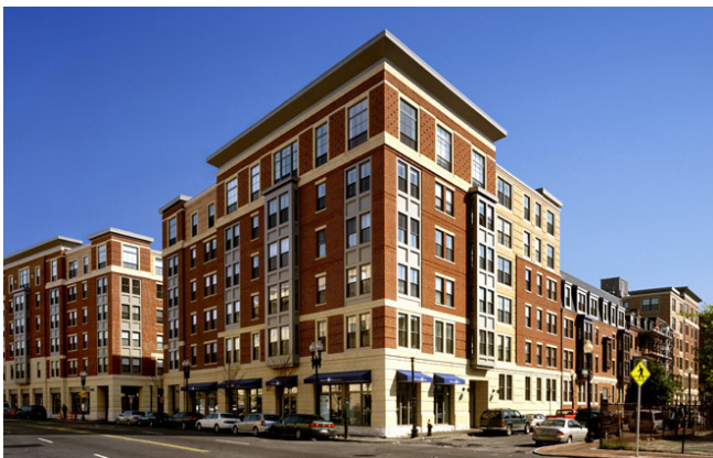
C.4-03: Transitional design combines historic and contemporary elements, producing buildings sympathetic to a traditional context. Decorative articulation is often present in the form of stringbands and cornices, albeit in stylized or abstracted form.
