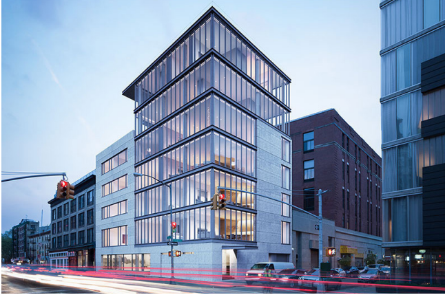
C.4-10: Modern design, with a typically narrow palette of minimally-detailed materials and emphasis on abstract form, can take on contextual qualities and visual interest through overall massing and contrasts between solid walls and glazing.
