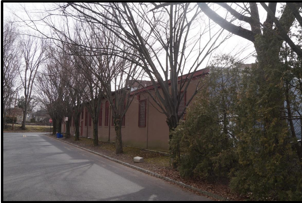
PLATE 10: 6-10 ERIE STREET. VIEW SOUTHEAST. WIECZOREK: 2/16/2023.
