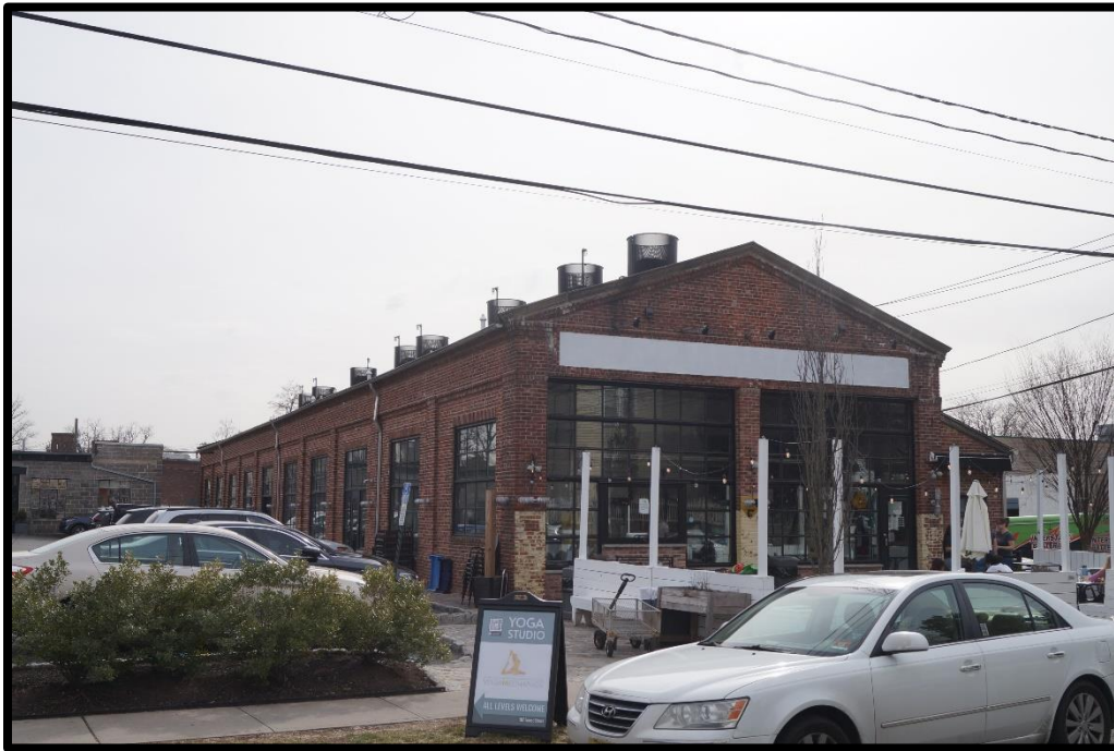
PLATE 1: 16 LABEL STREET. VIEW SOUTHEAST. WIECZOREK: 2/16/2023.
