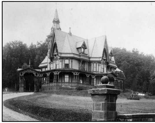
Figure 18. Samuel Crump's Residence on Highland Avenue. Demolished. P2933 Montclair Public Library Photo Database.
