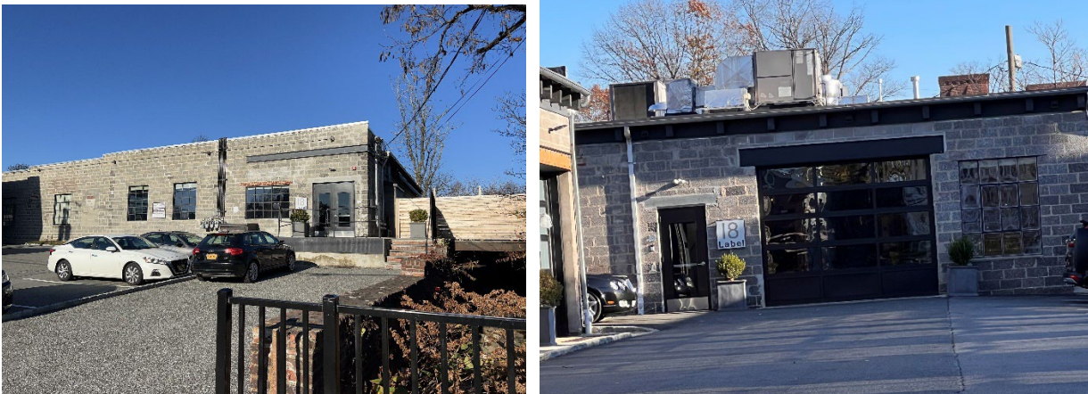
Industrial Building – 1950 – possible Oiljak Company
