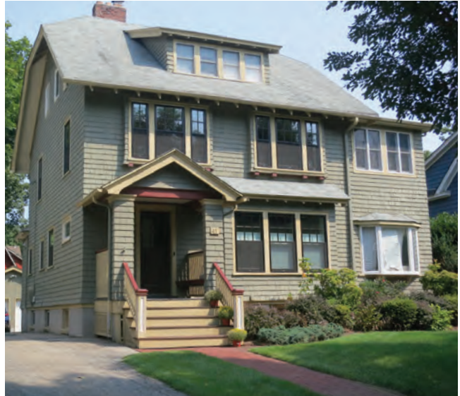
Shingles, deep eaves, grouped windows in projecting bays, window shed, decorative beams under the gables and a low-pitched porch create a Craftsman composition.
