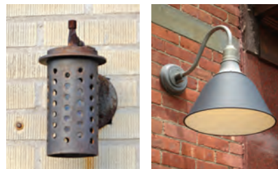
Dark sky fixtures are available in many styles & limit upward and stray light pollution.
