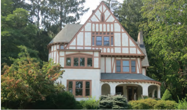
Steeply pitched roofs, multi-paned glazed windows and decorative half-timbering identify the Tudor Revival.
