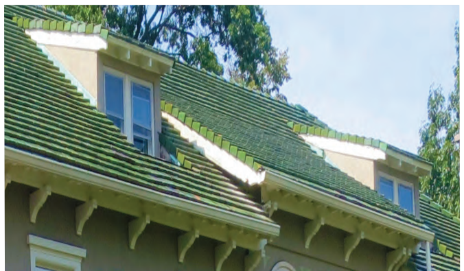
Check original manufacturers and architectural salvage sources online for replacement historic terra cotta tiles like the green units shown here.
