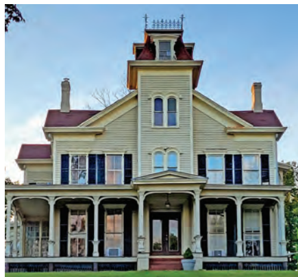
A generous wraparound porch provides a graceful base for walk-through windows and a flared Mansard roof.
