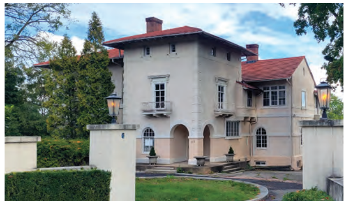
The former home of 19th century sculptor William Couper was designed by A. F. Norris in 1905. a local architect. Known as “Poggioridente”, it was featured in “Concrete & Country Residences”, 1906, Portland Cement Company and is listed on the National and State Registers.
