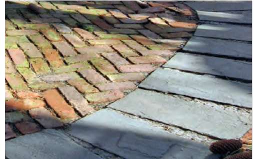
Below, flagstones and dry-laid bricks.
