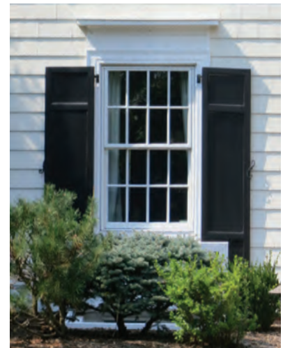
A projecting window head and operable shutters look good but can also serve their original functions of managing water running down or blowing at a facade.
