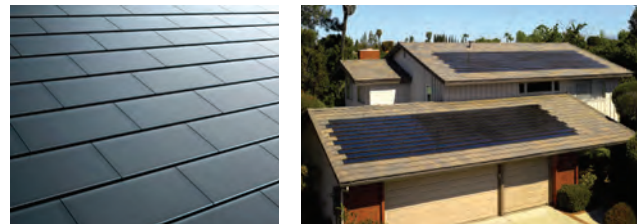
Building integrated solar like roofing tiles (left) and shingles (right) do double duty as roofing and power producer, as well as providing better looking installations.
