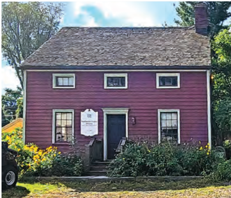
An intact New England style 3 bay side gable house.
