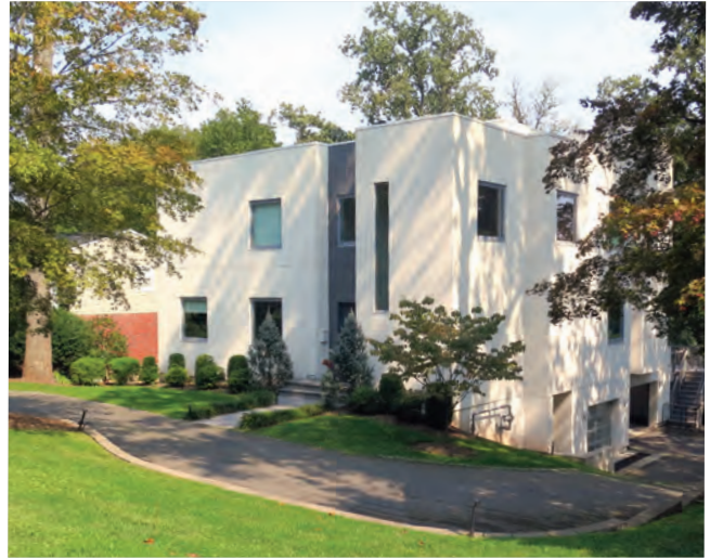
The flat roof, punched windows and unarticulated flat exterior surfaces are characteristic of much post-war modernism.
