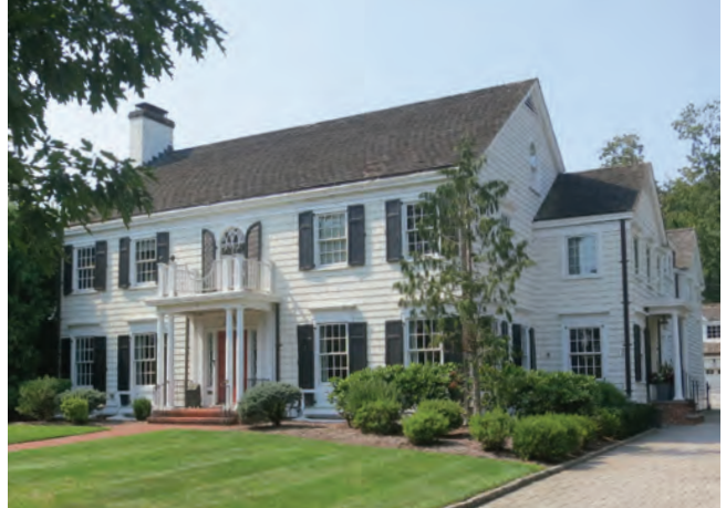
Details make this house distinctive: projected heads and shutters on full height windows, and the dialogue of arches between upper window and porch rail, above an elegant double columned entry.
