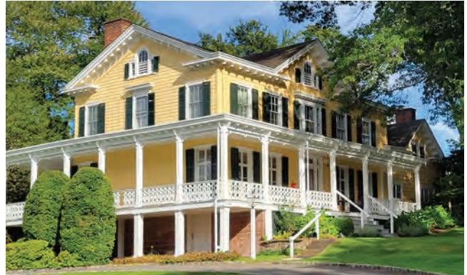
Low pitched roofs with decorative bracketed overhanging eaves and arched Palladian windows are characteristic of the Italianate style.
