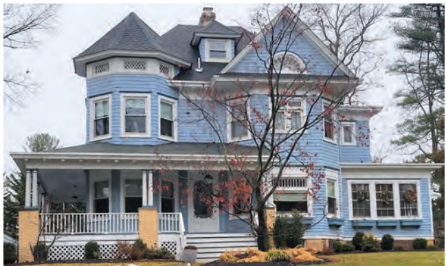
The octagonal tower with banded horizontal element and gable fanlight emphasize the asymmetrical façade of the Queen Anne style.
