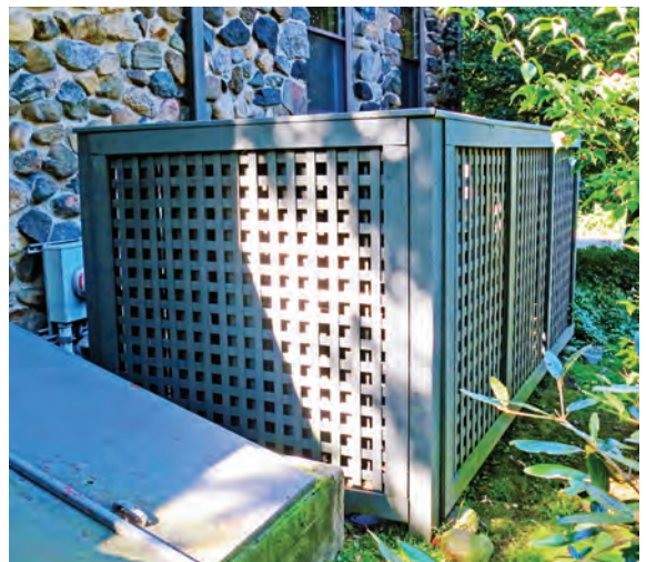
Air circulates through lattice enclosure hiding meter and air conditioning. Traditional square horizontal lattice is painted to blend with house palette.
