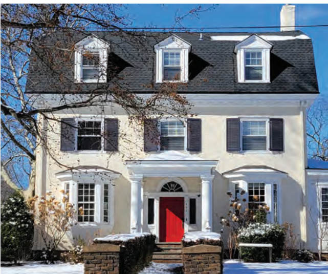
This Colonial Revival style house relies on symmetry in the window detail, correct shutter sizing and a dominant front porch with columned portico.
