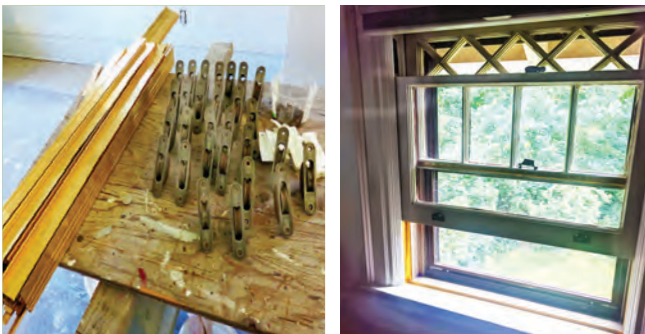
Preserving windows made of old growth lumber can save carbon. They can be made energy efficient and operational with a weatherstripping rehabilitation. Left: weatherstrips & pulleys. Right: finished window.
