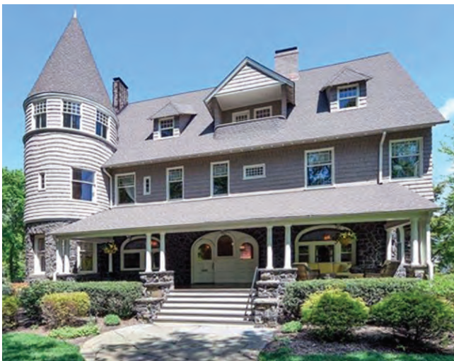
The rusticated stone foundation of the porch and tower, the rounded arches, double columns and decorative shingle composition express the Richardsonian Romanesque.
