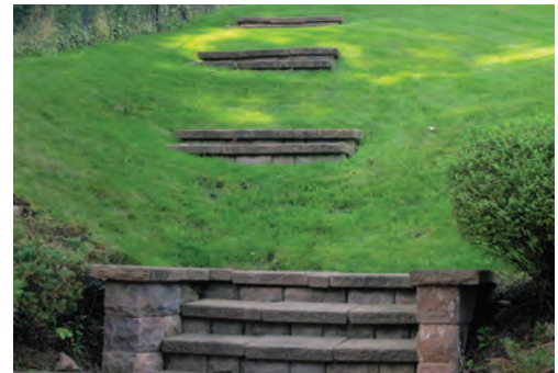
Perrons, or steps built into a hillside, can be a beautiful and less intense way of accommodating foot traffic.
