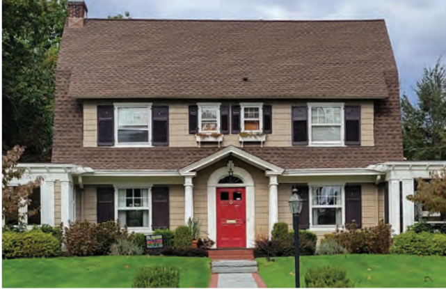
The gambrel or two-pitched roof originally appeared in Dutch American houses in New Jersey in the 18th century and became popular in the 20th century Dutch Revival because of the extra space it provided on the upper floors.
