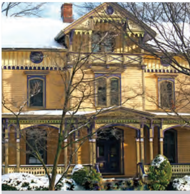
Stick style examples like this are memorable in the complexity of their virtuosic carpentry adornment, which often has see-through elements comprised of "sticking".
