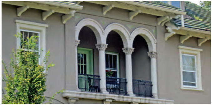
Stucco should allow trim to be expressed to create shadow lines and also manage water.
