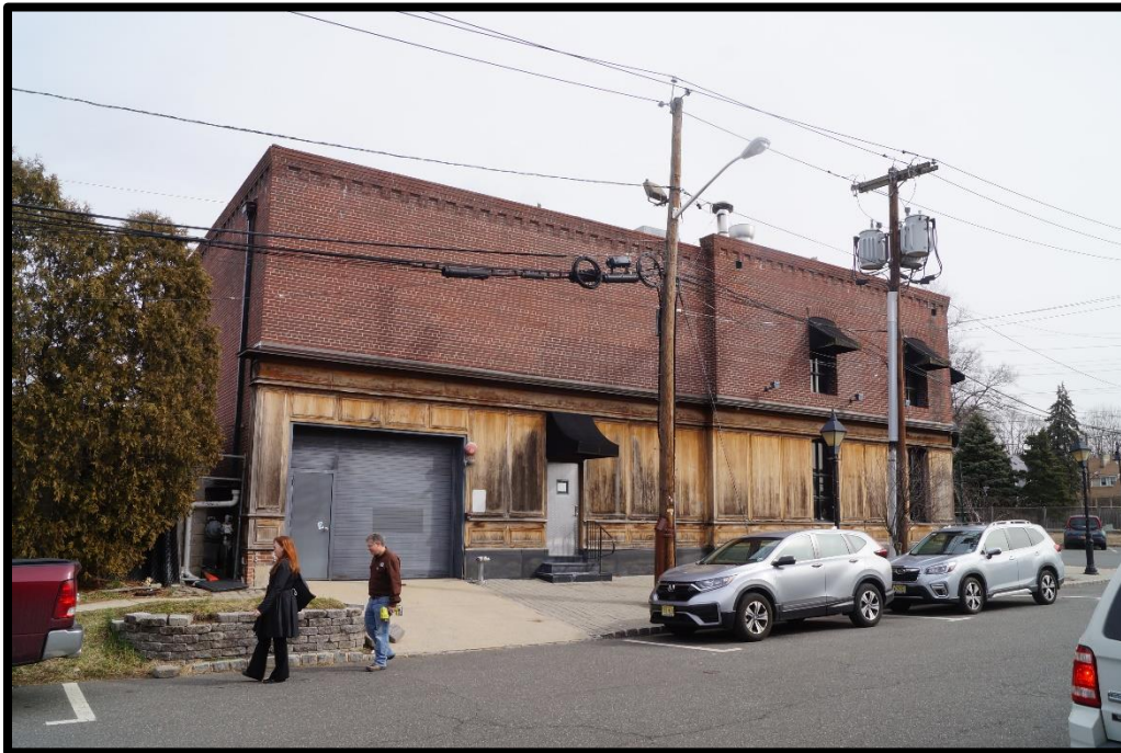
PLATE 6: 2 ERIE STREET, PART OF 6-10 ERIE STREET PARCEL. VIEW NORTH. WIECZOREK: 2/16/2023.
