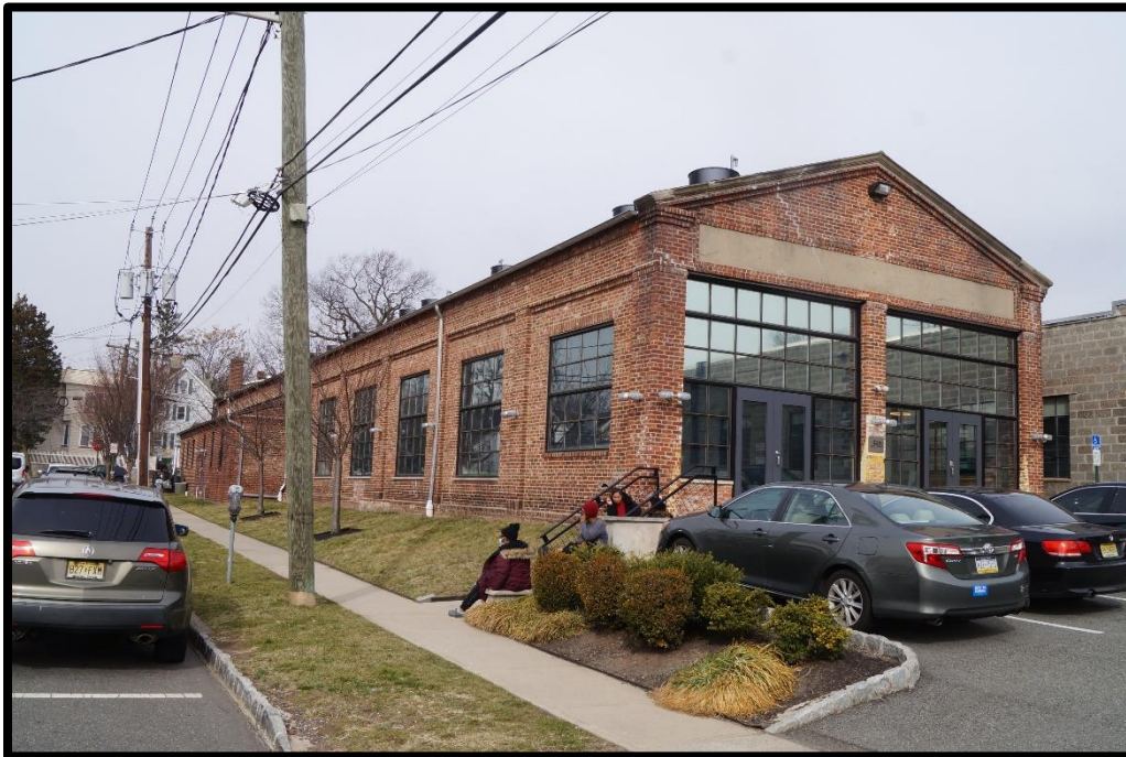
PLATE 3: 16 LABEL STREET. VIEW NORTHWEST. WIECZOREK: 2/16/2023.
