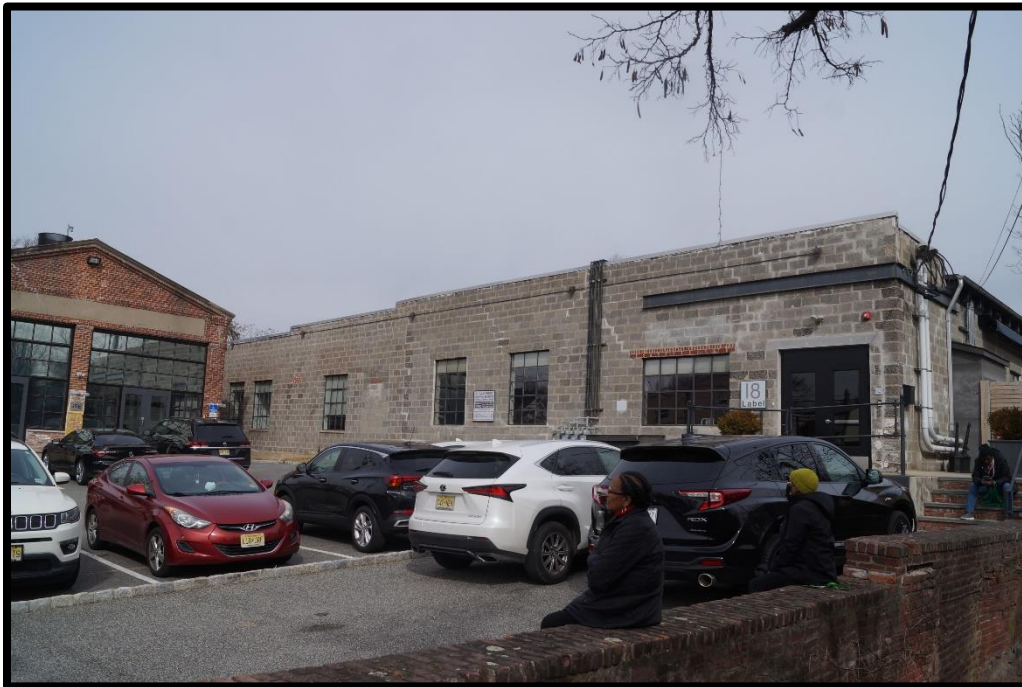
PLATE 4: 18 LABEL STREET. VIEW NORTHWEST. WIECZOREK: 2/16/2023.
