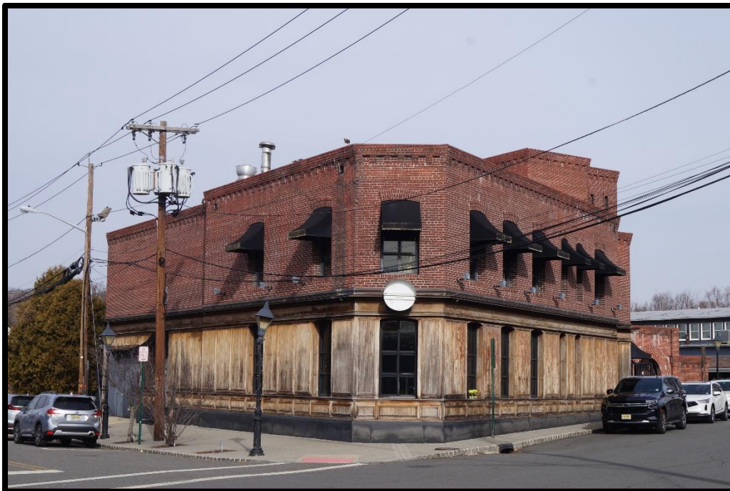
PLATE 5: 2 ERIE STREET, PART OF 6-10 ERIE STREET PARCEL. VIEW NORTHWEST. WIECZOREK: 2/16/2023.
