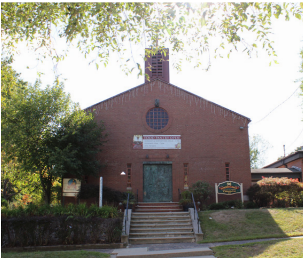
St. Peter Claver Roman Catholic Church (56 Elmwood Avenue, built c. 1939)
